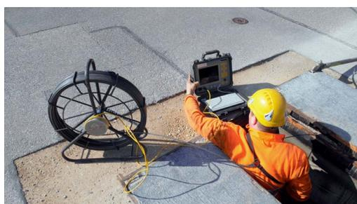
Probing the existing pipe system using a camera probe
