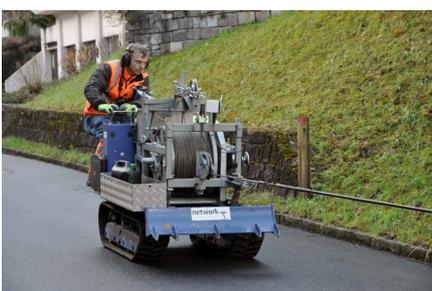
Cable feed using cable feed machine
