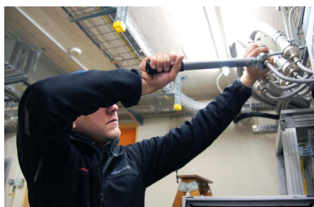
Connecting the antenna cables
