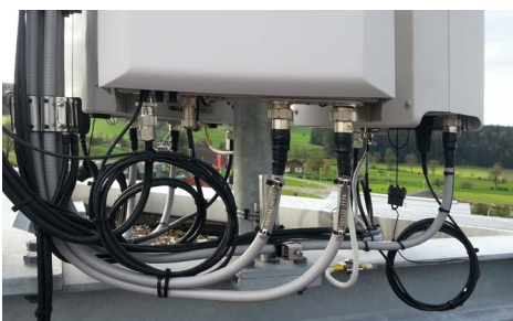
Wiring the RRU (Remote Radio Unit)
