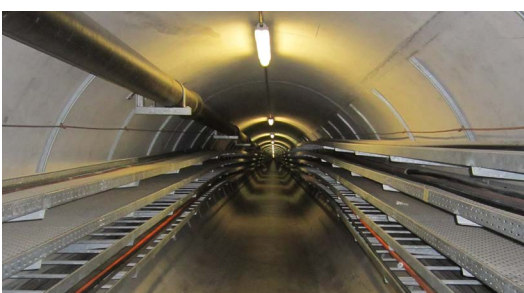
Ceiling installation of leaky feeder cable in the service tube
