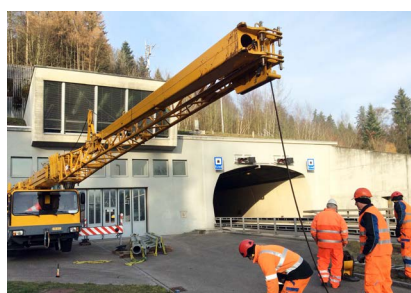
Setting up the Baregg Tunnel mast
